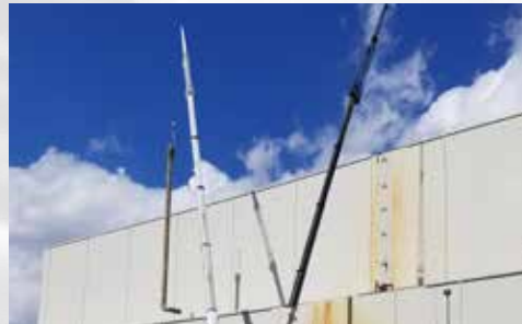
Provide pipe stress analysis, fabricate and field join a 70m vertical stack 🔄
