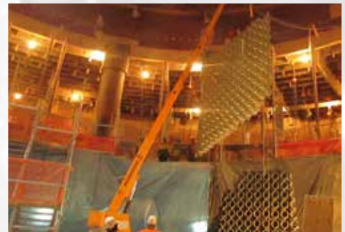
Lining of storage tank with 9' x 40' FRP panels 🔄
