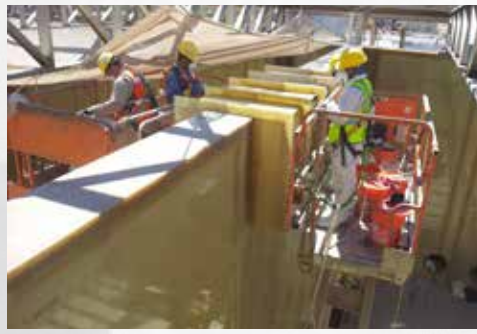
Provide pipe stress analysis, fabricate and field join a 70m vertical stack 🔄
