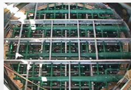
Design, fabrication and installation of wet scrubbers in FGD applications 🔄
