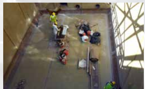
Lining of storage tank with 9' x 40' FRP panels 🔄
